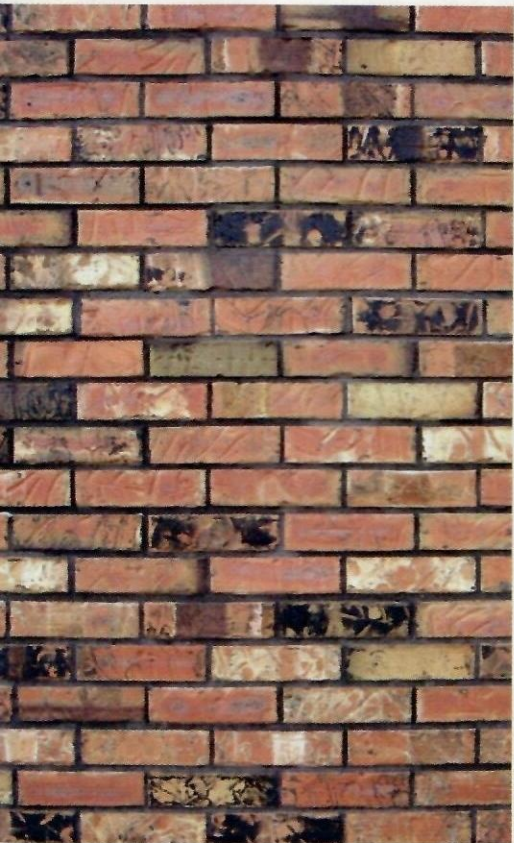
Concrete over bricks completed
